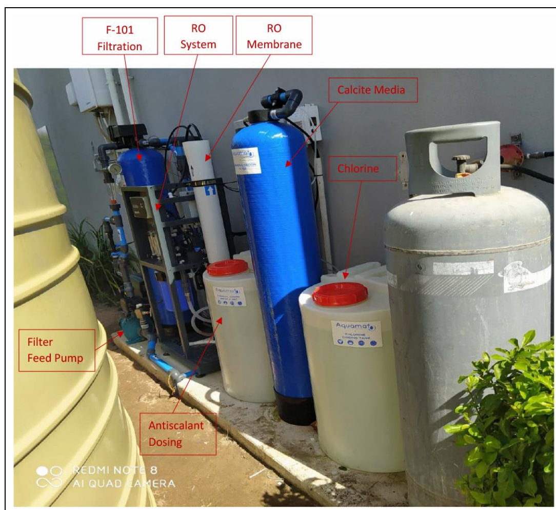
Illustration 5 – Proposed Water Treatment System.
