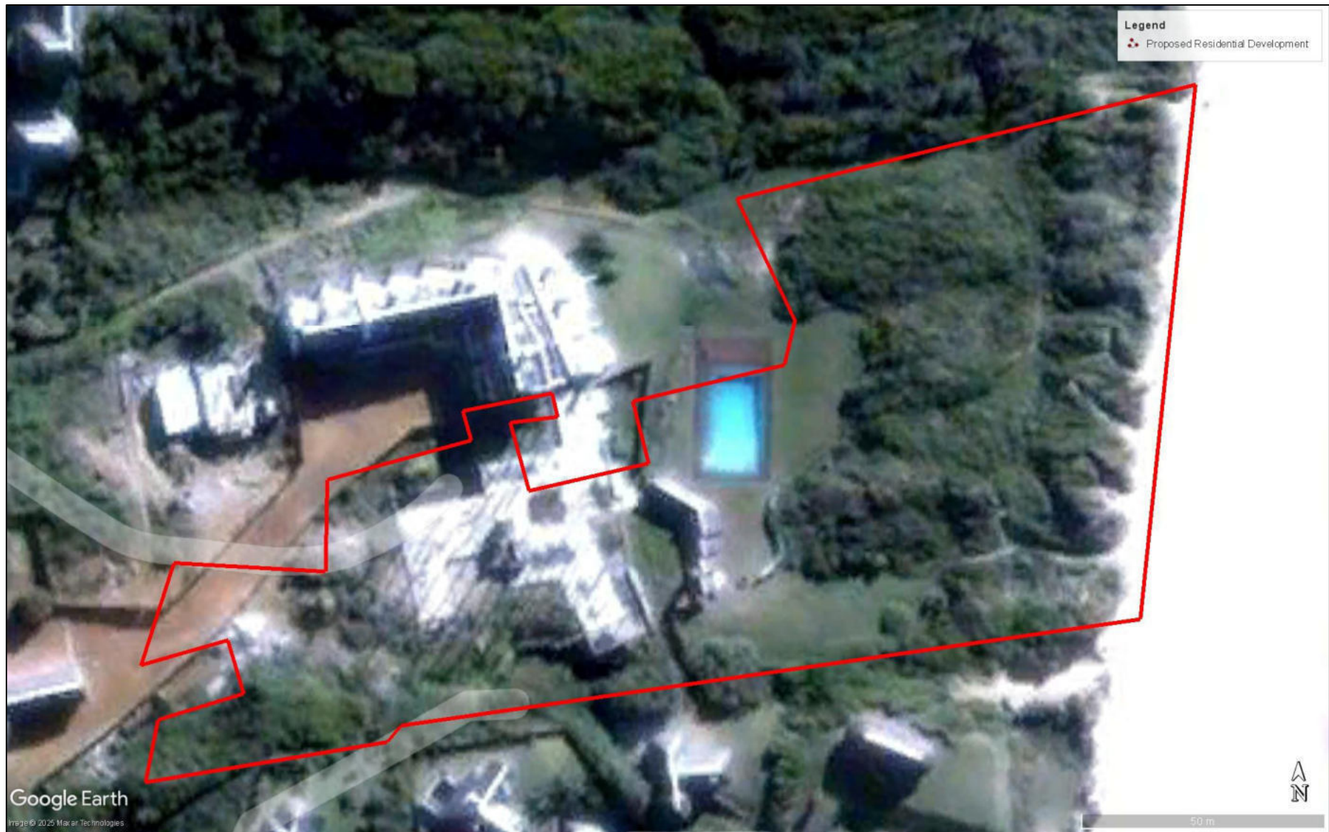
Figure 8. Close up of the proposed residential development and the ruins of the existing built environment structures (historical – years 2002/2003).
