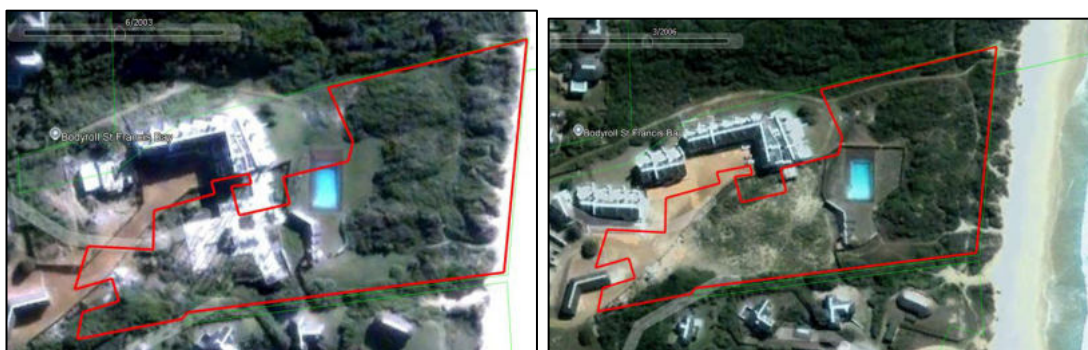
Figure 1: The hotel in 2003 burnt down sometime between 2003-2006, as Google Earth shows that most of the Hotel structure is gone, however onsite photos indicate that foundations was never removed.
