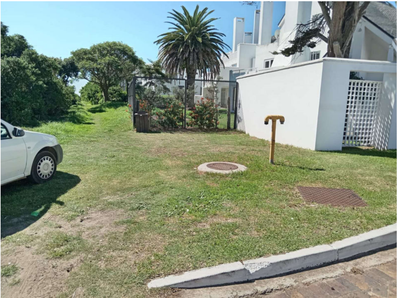
Figure 6: Booster connection and sewer manhole in Diana Crescent.
