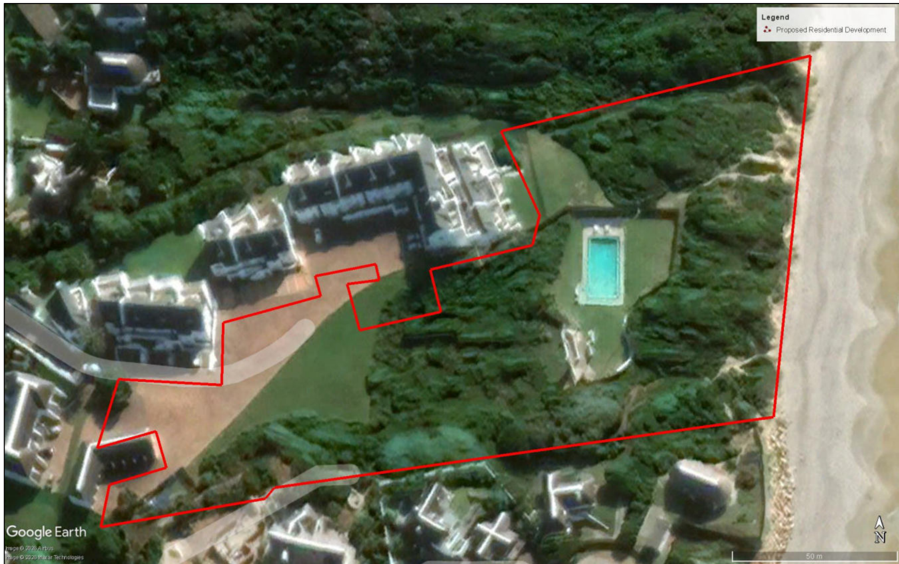
Figure 7. Close up of the proposed residential development and the ruins of the existing built environment structures (current – 2026).
