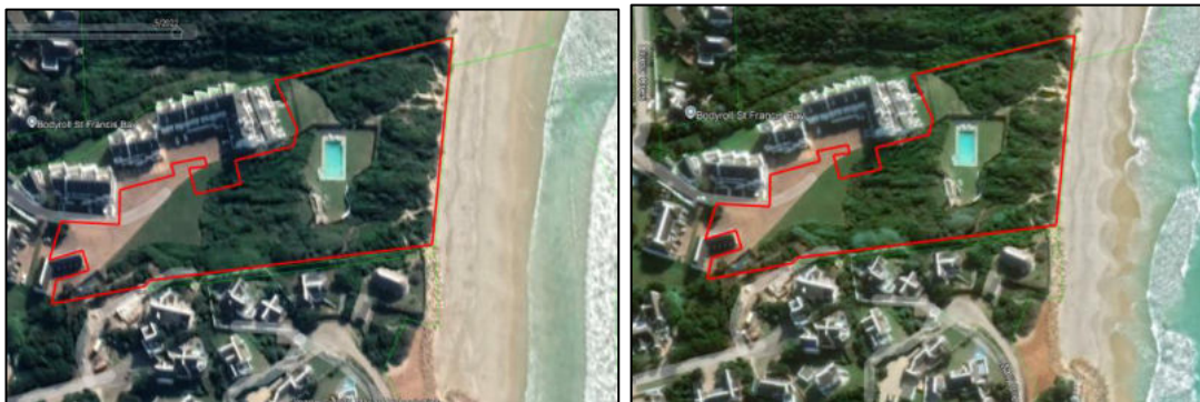
Figure 3: In 2022 the erosion control along the coastline increased further southwards.
