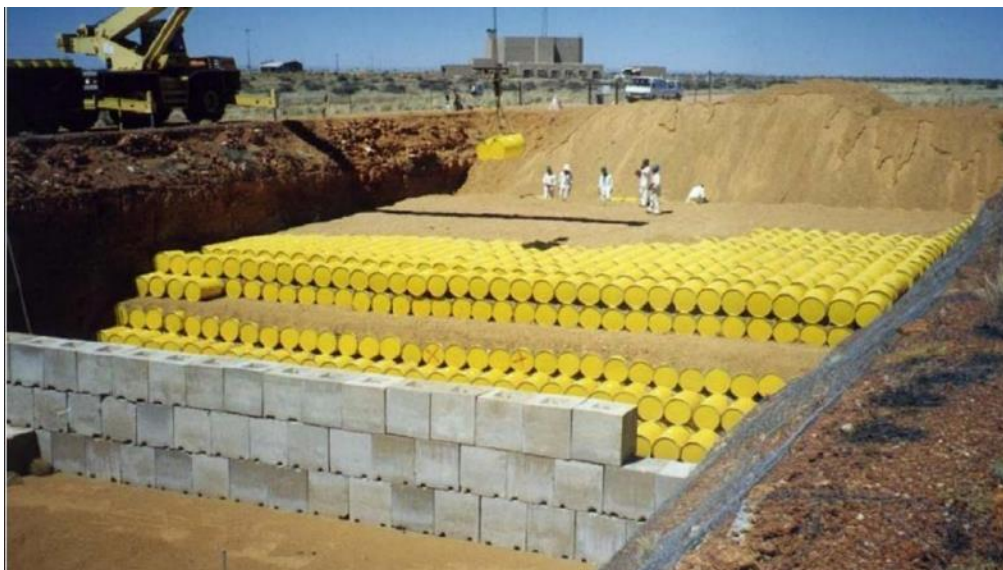
Figure 4-3 – Storage of Waste at Vaalputs Nuclear Waste Storage Facility
